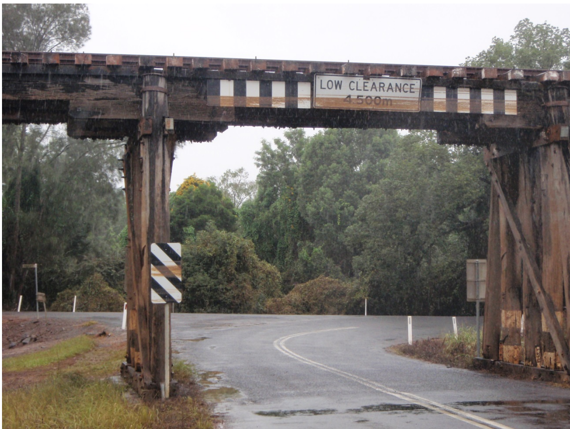
Wilson's River, Winterton Parade North Lismore 12.39pm 4 April 2017 debris line on bridge
